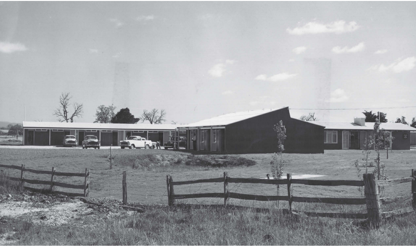
John E. Jansson, photographer, [View from boundary fence of the exterior Mitchell Valley Motel Princes Highway Bairnsdale]. C. 1959. Pictures Collection, State Library of Victoria [H2013.188/7/2]
