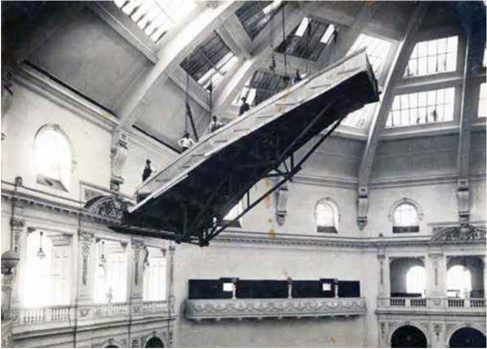
Above: Men on a suspended scaffold, said to be for repairs to the glass skylights, c. 1918, but more probably for the lining work. Photo by Sutcliffe Pty Ltd. SLV, H36621.
