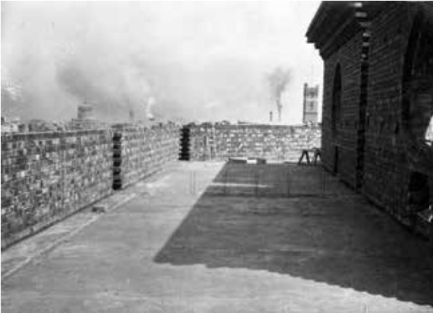
Above: View along the south-east side of the annulus roof, with projecting rods designed to tie into the brick buttresses: Clark photos, State Library of Victoria, H93.39/33. The altered buttress design, 'Alteration to walls at roof level [Domed Reading Room, Melbourne Public Library] / Bates Peebles & Smart. Annotated in red crayon and black ink l.l.: Kindly Return / to W W Harvey / c/- Thos Cook & Son / Ludgate Circus / London. Annotated in black ink l.r.: Recd 25.5.10 / WWH. SLV, H2010.69/78. Below: Concreting a 21 x 24 inch [525 x 600 mm] beam under a roof buttress. Clark photos, SLV, H93.39/126.
