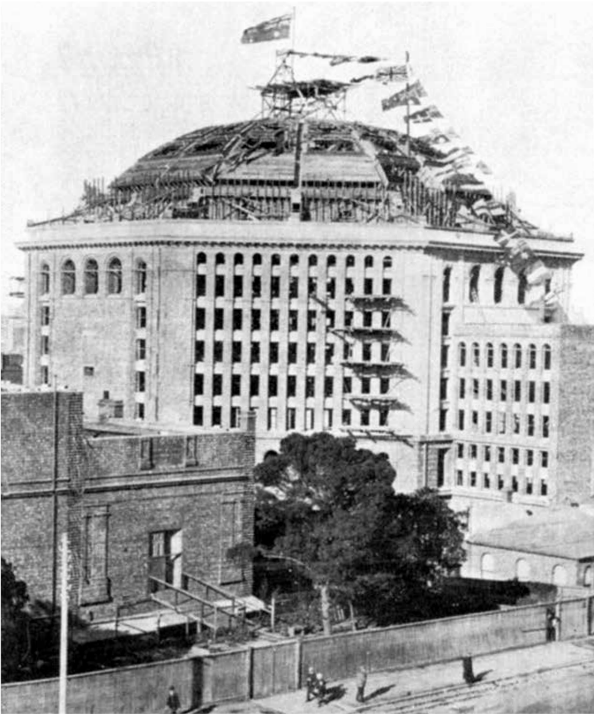
The dome decorated for the completion of the formwork. Building , 12 June 1911, p.53.
