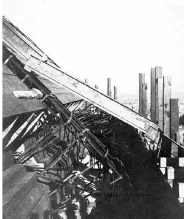
Above: Constructing the base of the dome c. 1911, with the Kahn reinforcing bars visible, Clark photos, SLV, H93.39/28, H93.39/30.
