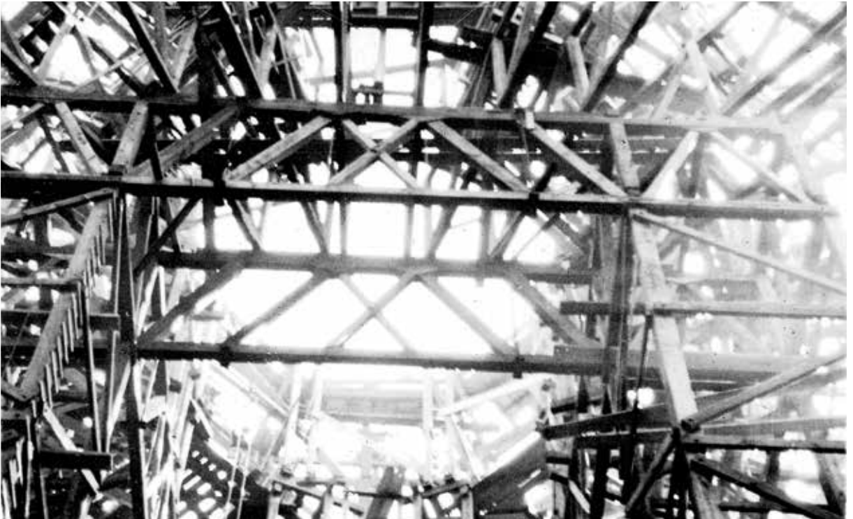
Below: 'Towers etc. [and] dome centering', 1911. Clark photos, SLV, H93.39/23.
