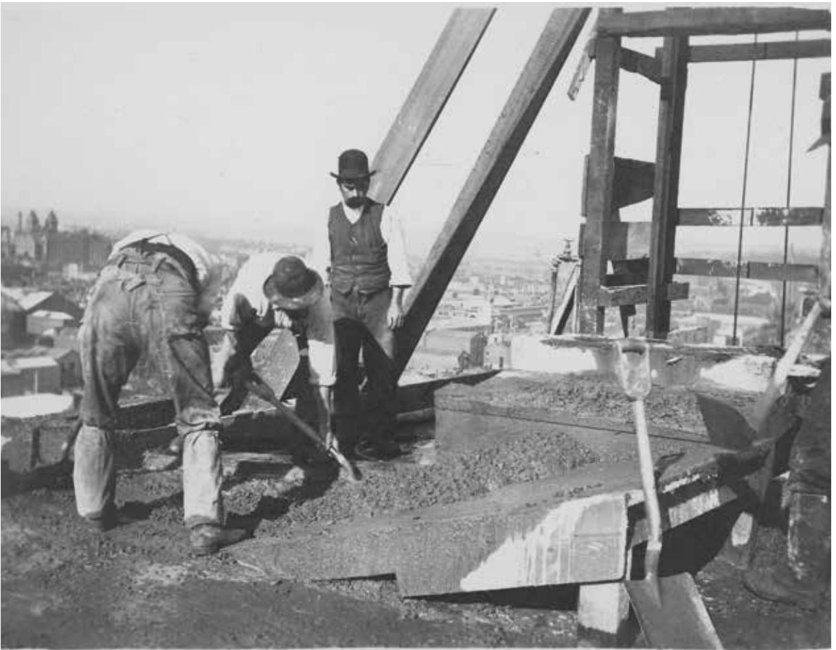
Laying concrete on the roof of the annulus corridor, c. 1910. J. R. T. Clark, foreman in charge of the concreting, standing at centre in waistcoat and bowler hat. Clark photos, SLV, H93.39/27
