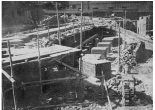
Above: Brick footings at for the octagon wall, c. 1909. Clark photos, SLV, H93.39/2; H93.39/4. Top: Excavations at basement level, prepared for the pad footings of the stanchions. c. 1909. Clark photos, SLV, H93.39/1; H93.39/5.
