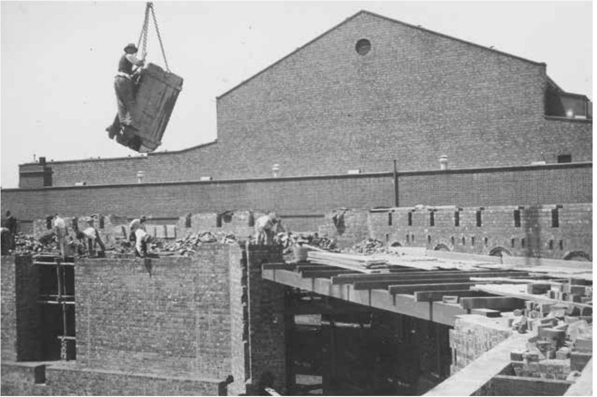
Above: Looking east at first gallery level 1909. Clark photos, SLV, H93.39/15.
