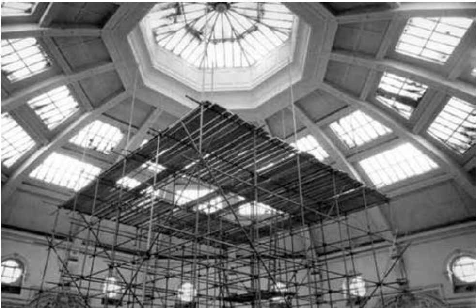
Below: Scaffolding of the Reading Room, 27 June 1958, photo by C.A. McCallum, Chief Librarian, SLV, H40298.
