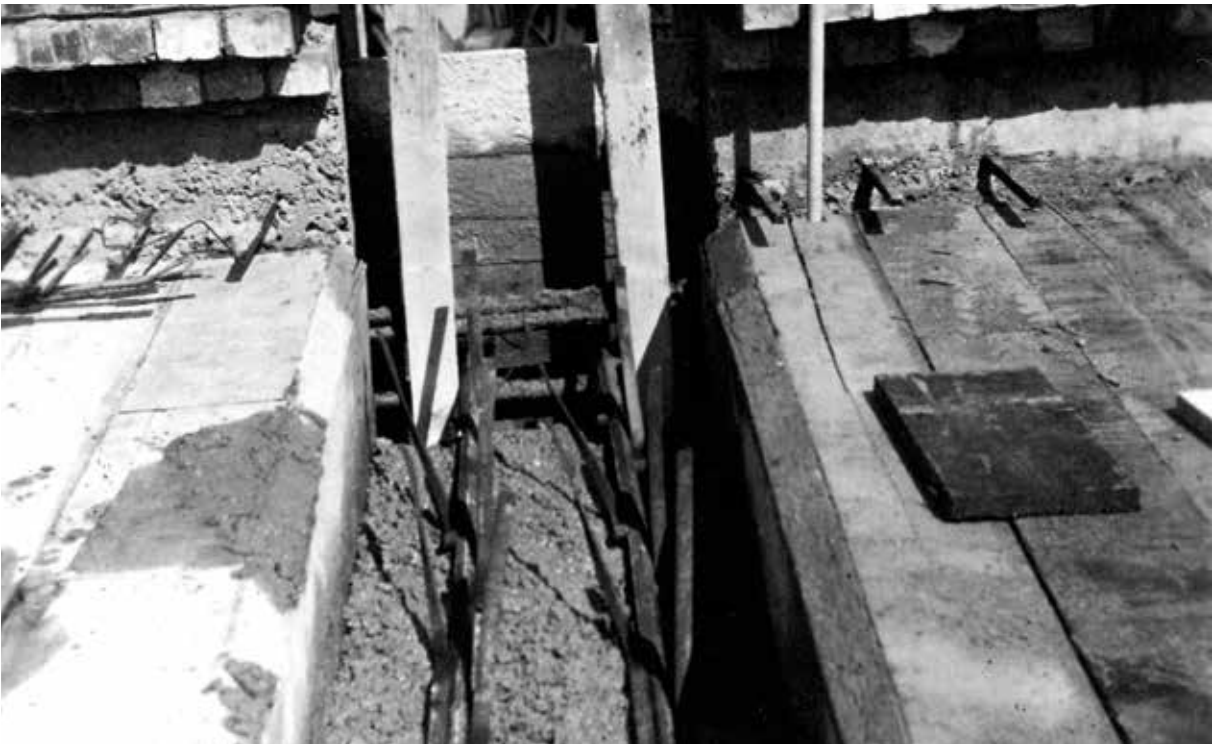
Above: View along the south-east side of the annulus roof, with projecting rods designed to tie into the brick buttresses: Clark photos, State Library of Victoria, H93.39/33. The altered buttress design, 'Alteration to walls at roof level [Domed Reading Room, Melbourne Public Library] / Bates Peebles & Smart. Annotated in red crayon and black ink l.l.: Kindly Return / to W W Harvey / c/- Thos Cook & Son / Ludgate Circus / London. Annotated in black ink l.r.: Recd 25.5.10 / WWH. SLV, H2010.69/78. Below: Concreting a 21 x 24 inch [525 x 600 mm] beam under a roof buttress. Clark photos, SLV, H93.39/126.
