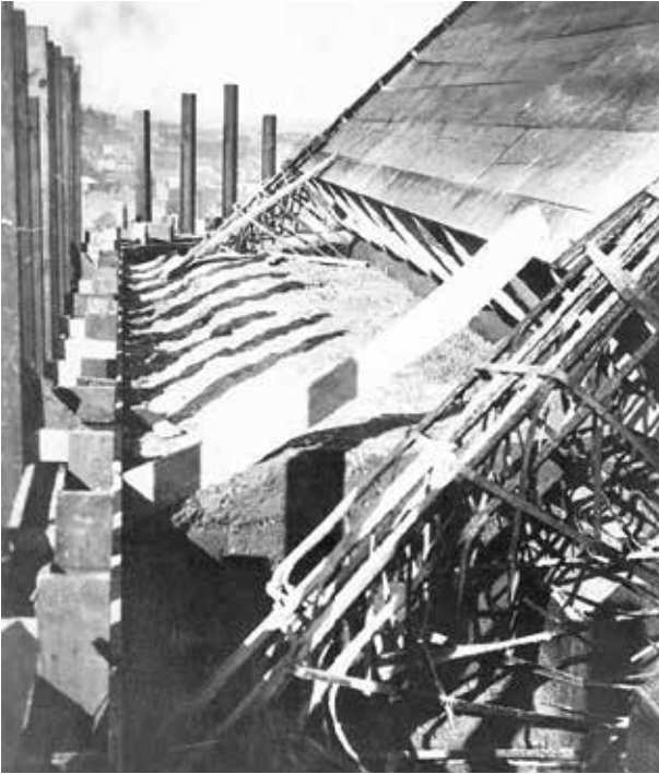
Above: Constructing the base of the dome c. 1911, with the Kahn reinforcing bars visible, Clark photos, SLV, H93.39/28, H93.39/30.
