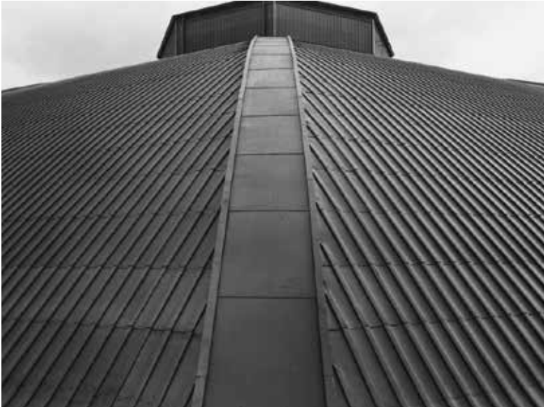
Copper cladding of the dome by Specialised Building Services Pty Ltd of Moreland, 1959. Photo by Wolfgang Sievers. SLV, H2001.172/1.
