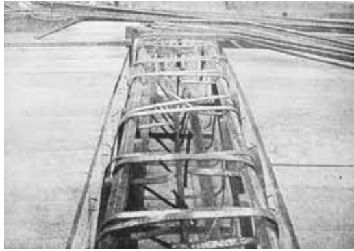
The Kahn reinforcement in place in the main floor beams. Truscon: the First Fifty Years: a short history of The Trussed Concrete Steel Company Limited, 1907-1957 (London: Truscon House, 1957), p 7.
