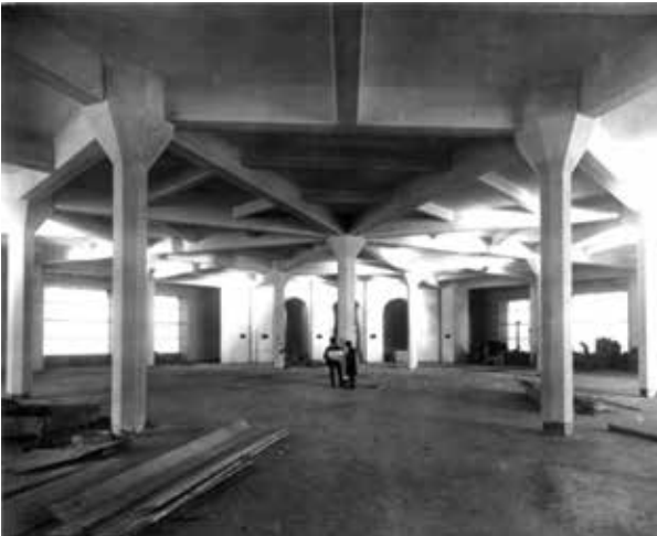
Left: The ground floor as constructed. SLV, H9217. Right: Dennys Lascelles Austin & Co Wool store, Clare, Corio & Brougham Streets, Geelong, by E. G. Stone (1909) 1910-11, with a clear span of 53 metres (the props were modern, and proved superfluous). Demolished 1990 at the instigation of the Cain Labor Government.
