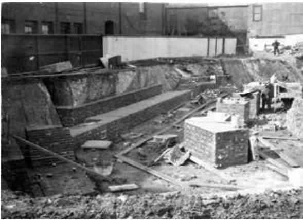
Above: Brick footings at for the octagon wall, c. 1909. Clark photos, SLV, H93.39/2; H93.39/4. Top: Excavations at basement level, prepared for the pad footings of the stanchions. c. 1909. Clark photos, SLV, H93.39/1; H93.39/5.
